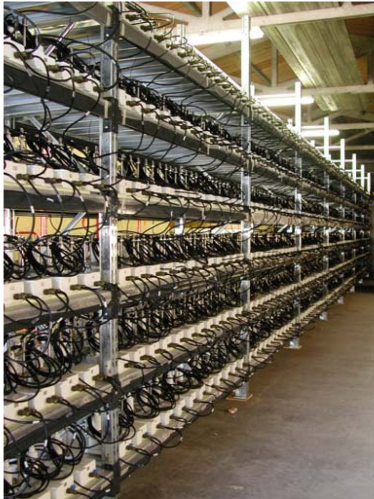
Fig. 2.2 1116 actuators network for SRT
