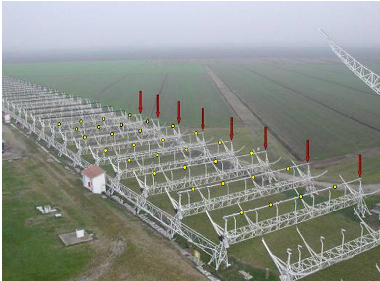
Figure 4: BEST-2 section of the Medicina Northern Cross Radiotelescope, courtesy of Marco Schiaffino
